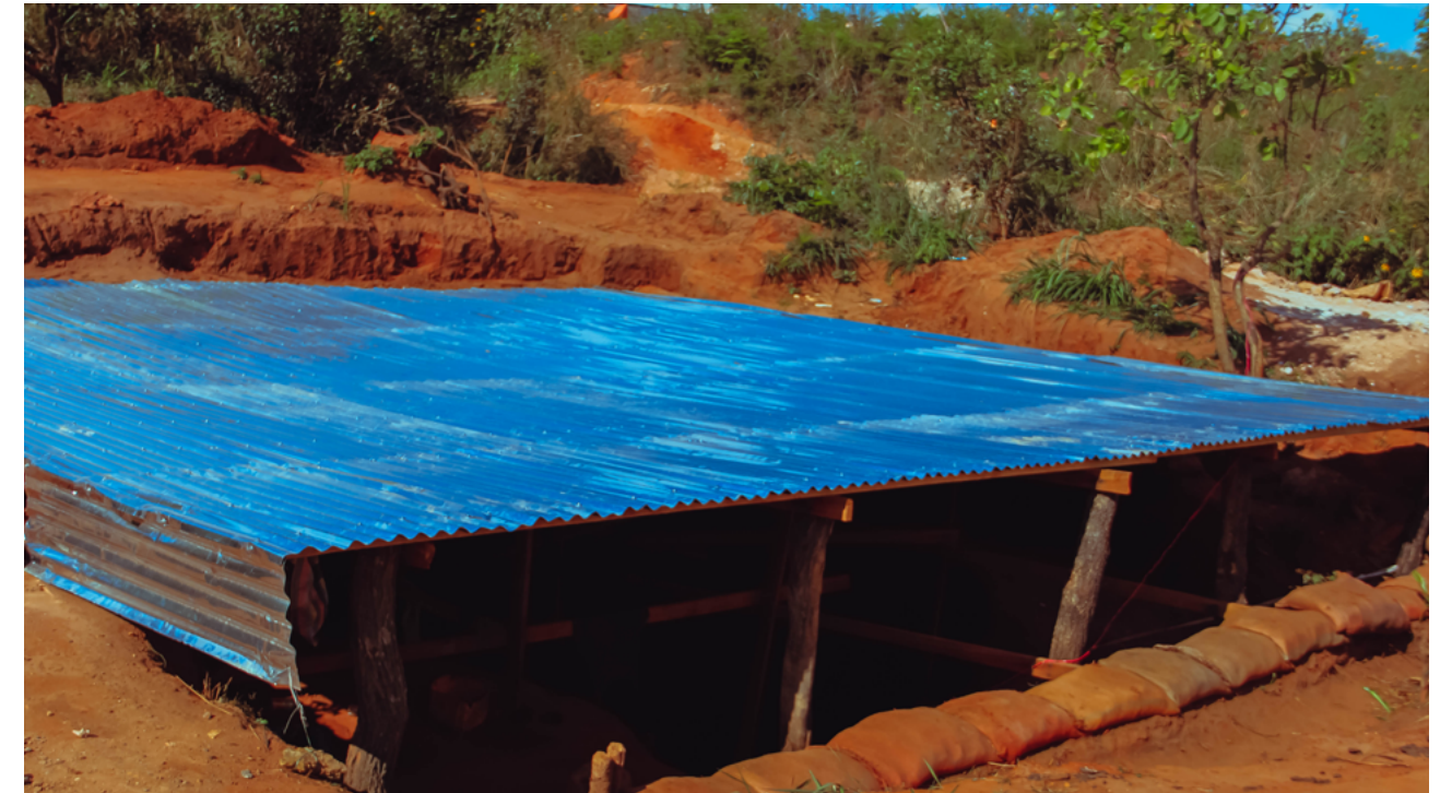
A pit recently covered with iron sheets – a durable alternative to the tarpaulins commonly used – to prevent accidents such as falling rocks and other hazards, such as flooding when it rains.
