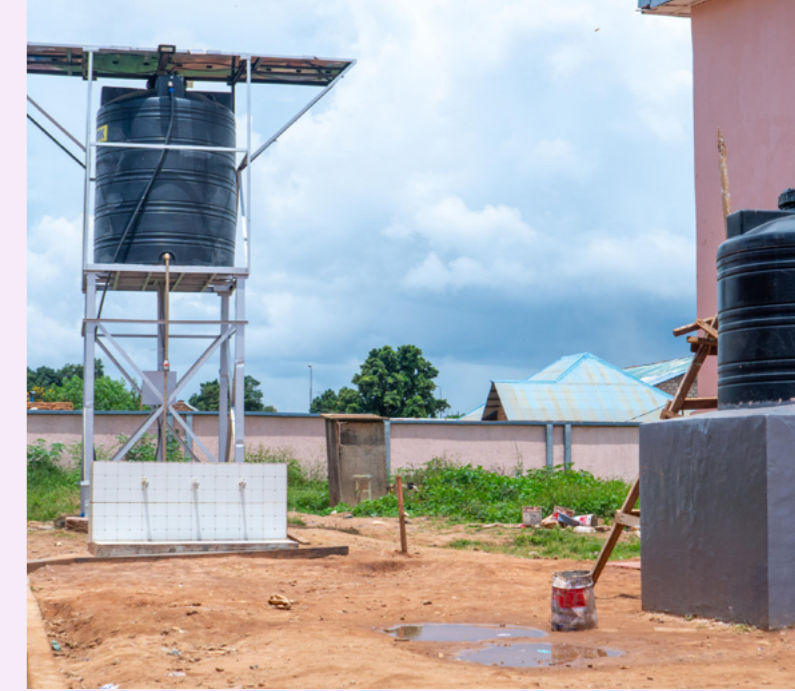
Drilled well at Dima Primary School.
